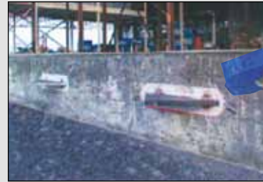
Diamond Dowel for slabs on the Ground
