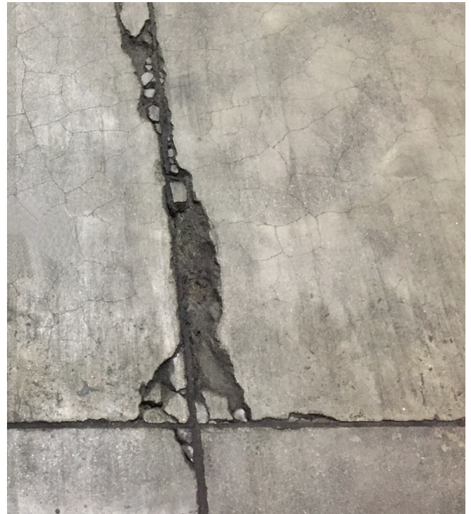
Joint damage
