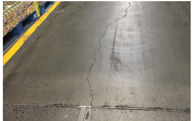
Cracks in Floor
