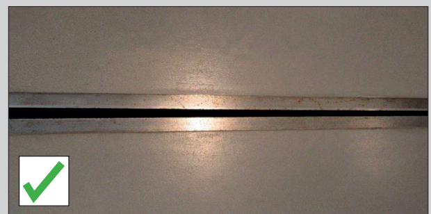
Installed Viper Joint
